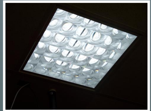
Solar Tube Light Fixture
