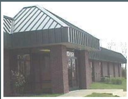
OVEC Offices in Shelbyville, Ky
